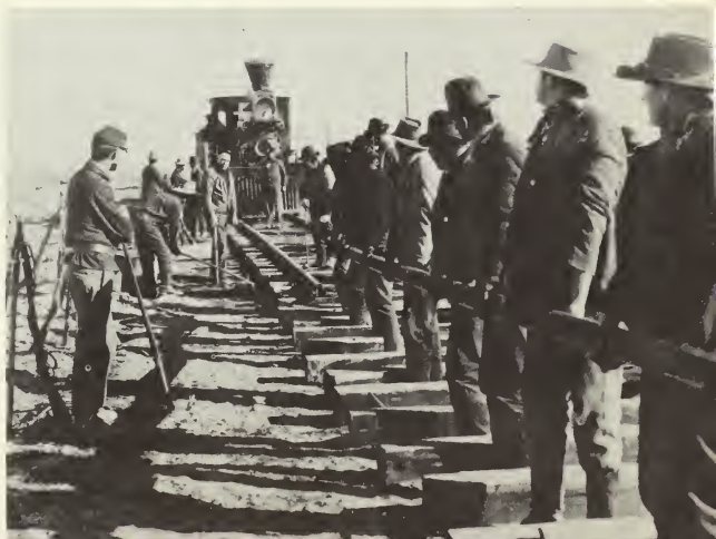
The track-laying race in The Iron Horse.
